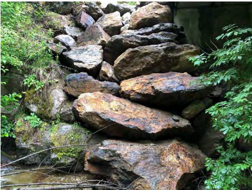
Upstream left bank riprap
