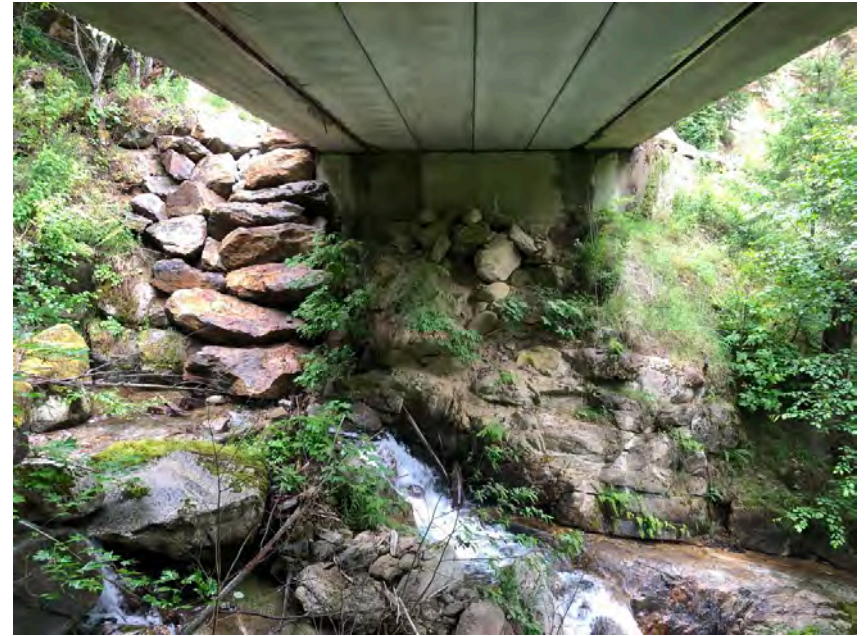
Left Bank Abutment when facing downstream
