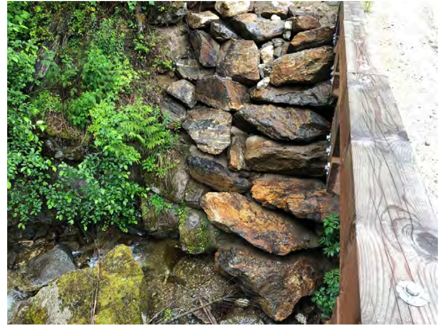
Upstream right bank riprap
