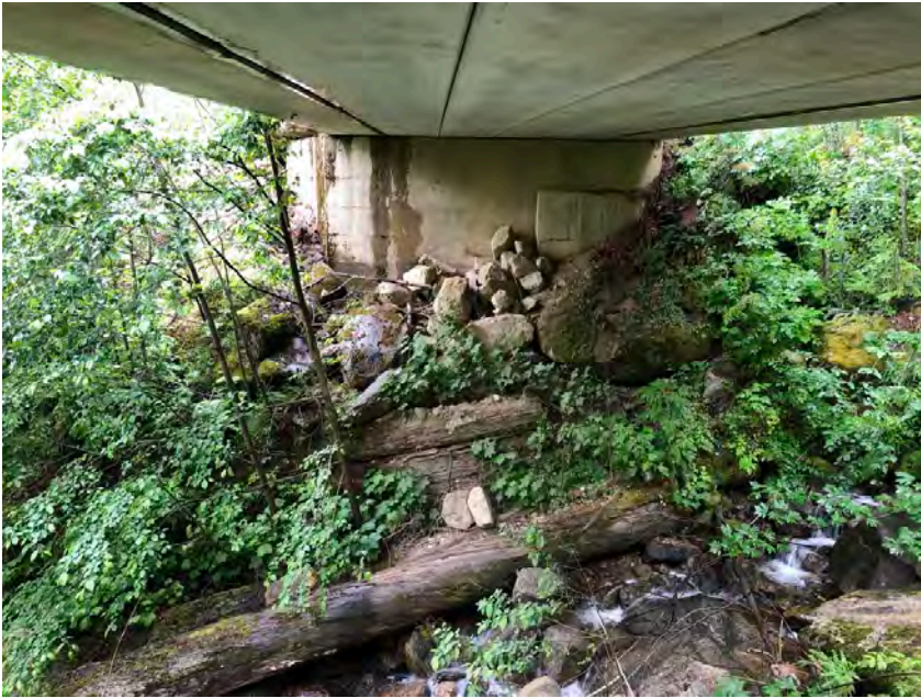
Right Bank Abutment when facing downstream
