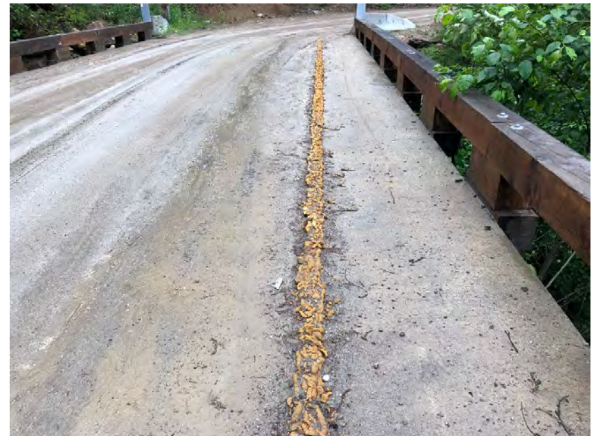
Spray foam used to fill joint on outside slabs
